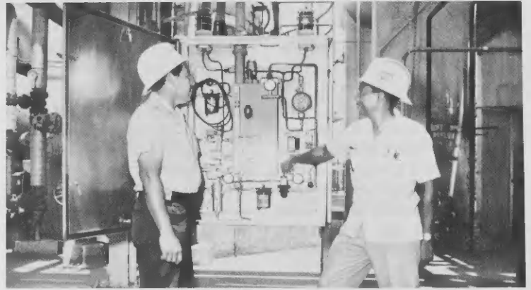
Pedro Tromp (at left) and Ramon Hodge adjusting the oil mist generator distribution pressure.
